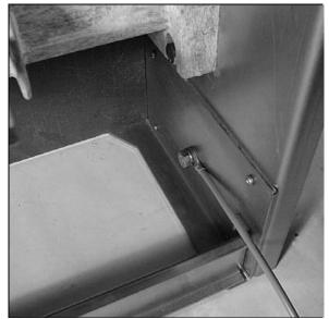
Fig. 14 Installation of Ground Wire
